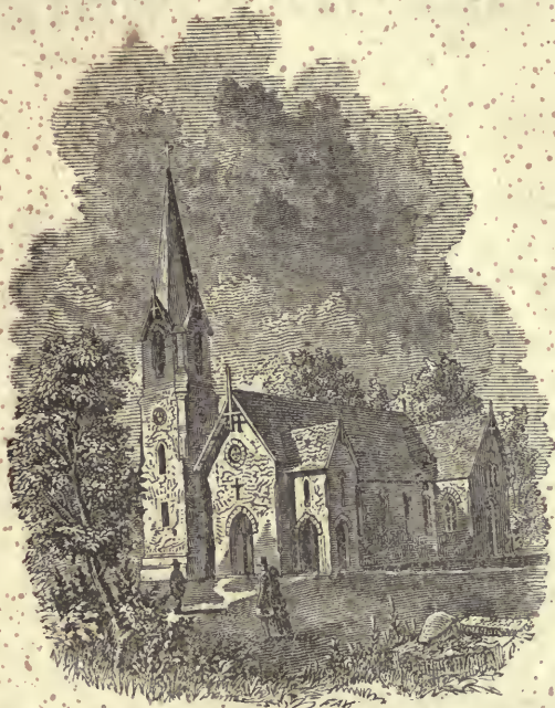
St. Peter's Church, Westchester—Erected A. D. 1855.
